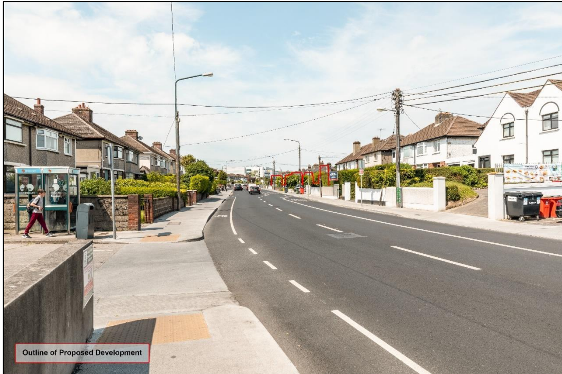
View 14.13: From Swords Road (R104), looking north towards the subject site
