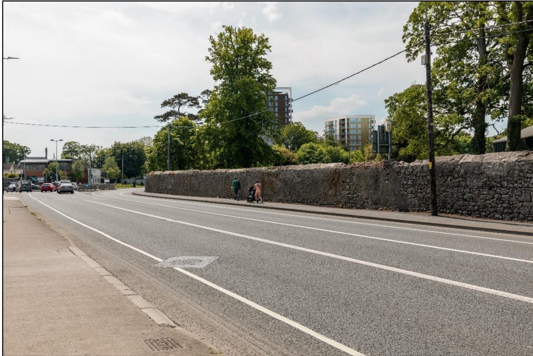
View 14.5: From Swords Road (R104), looking south towards the subject site
